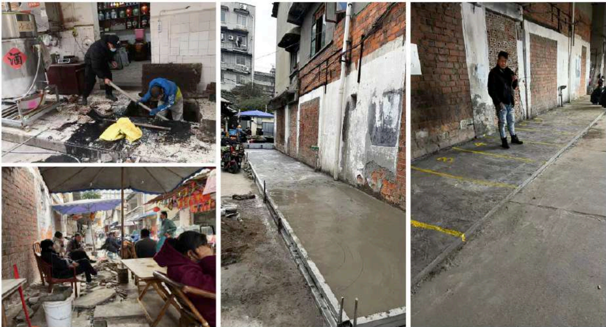
Fig. 6-10 Renovation of sewerage and pavement; the yellow line of vending unit
