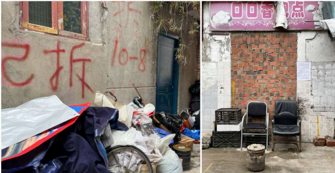
Fig. 6-16 The text painted on the wall “yi chai” (yi - already; chai - demolish); bricked shopfront on the street.
