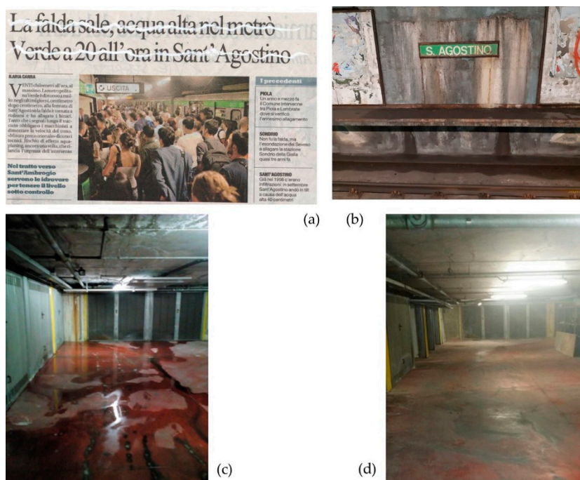
Figure 12. (a) Newspaper article of “La Repubblica” (2 July 2013), dealing with flooding episodes in Sant’Agostino station. (b) Flooding evidence in Sant’Agostino station (8 September 2020). (Image credits to the authors). (c) Flooding evidence in Numa Pompilio public car park. (d) Absence of flooding evidence after waterproofing works in Numa Pompilio public car park. (c,d): images were provided by Rete Irene.
