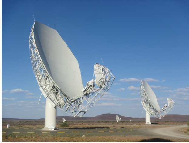
Figure 7.1: Close up picture of a MeerKAT antenna. Credits: SARAO
