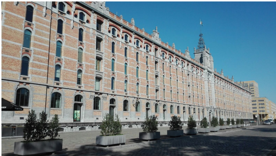
Figure 3-6: the Tour and Taxis Site
