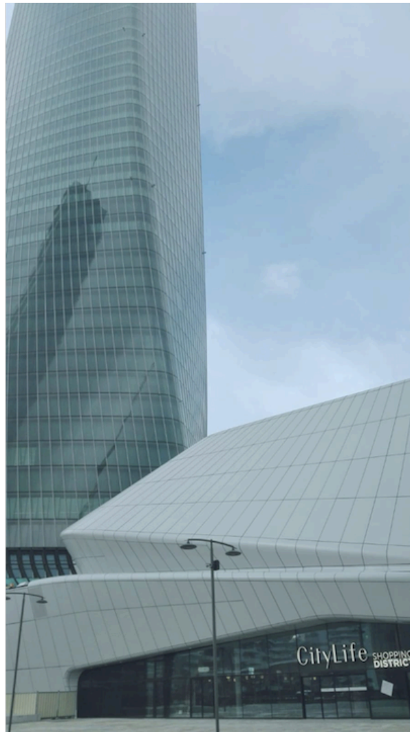
Figure 4-10: The shopping mall and the tower by Hadid
