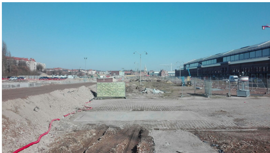
Figure 5-9: Construction works at February 2018
