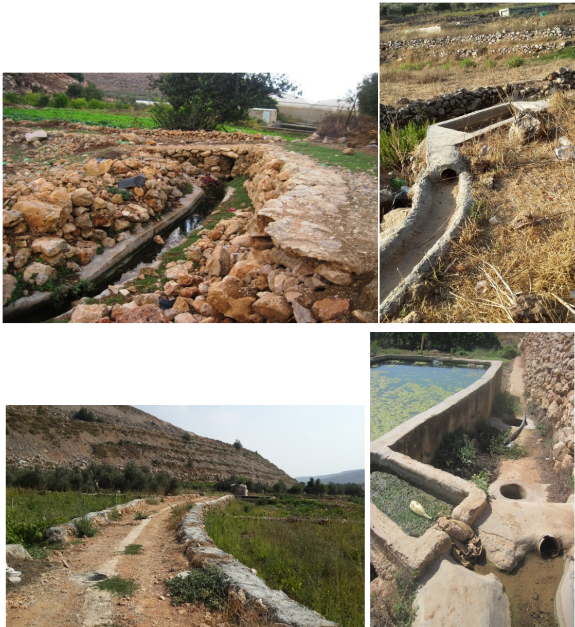
Figures 54, 55, 56, 57: open-air and covered concrete channels used for irrigation (De Donato 2016)
