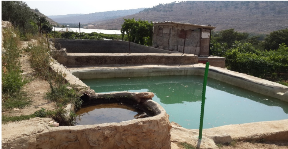
Figure 58: pools for the collection of spring water, used for irrigation (De Donato 2017)
