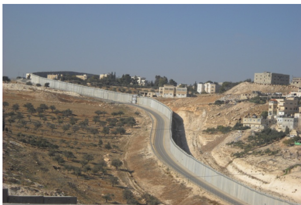
Figure 33: the Israeli segregation wall
