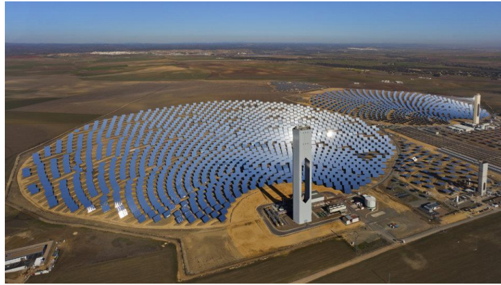
Fig. 1.1. Example of solar concentrator in Spain. The mirrors direct the solar energy onto the water tower. The water powers a steam turbine to produce electrical energy. 2
