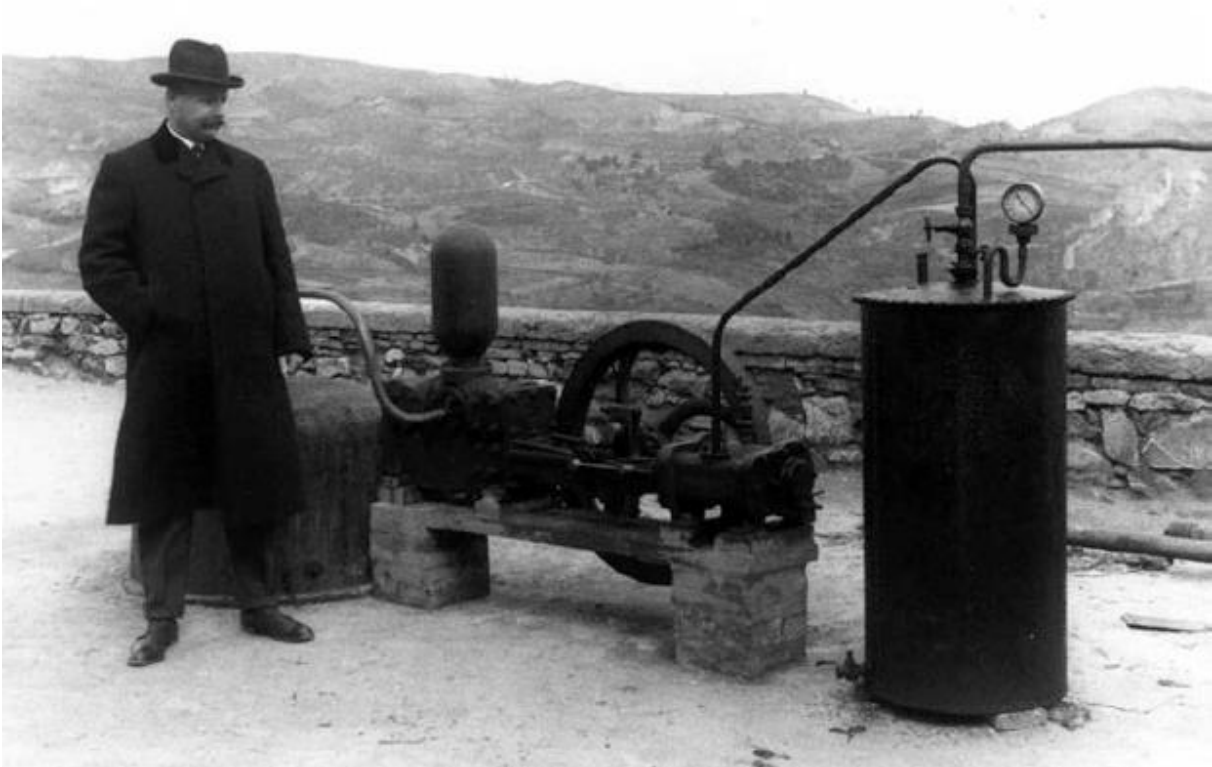
Figure 3.11: Lardarello 1904: The picture shows Principe Piero Ginori-Conti with his apparatus that converted geothermal to electrical energy for the first time in history. The installation had the power to light five light bulbs (Photograph: Unione Geotermica Italiana 2010).
