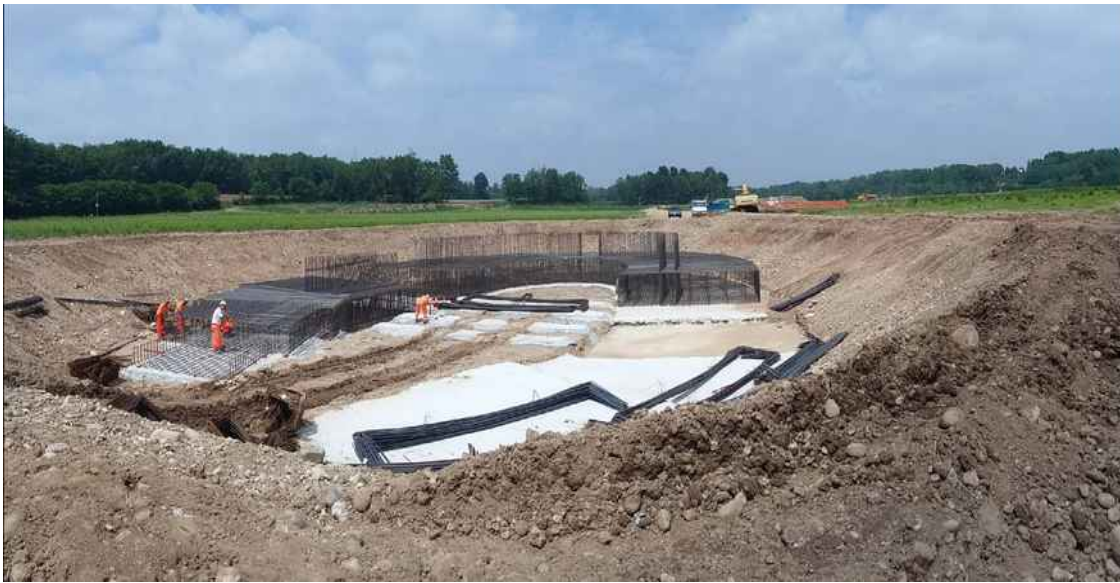
Fig.8.6 – Detention Basin under construction; source: Online
