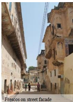
Frescos on street facade
