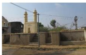
Historic water harvesting structures
