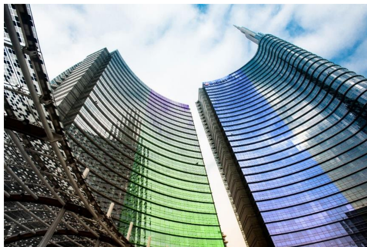
Figure 3.2.8: up, rendering of a Tesla Model S in which the windshield is made of an LSC sheet using subpc dimer as fluorophore. Down, rendering of Unicredit Tower in Milan showing the impact of covering the surface with LSCs based on DPP-Cy (left) and subpc dimer (right).
