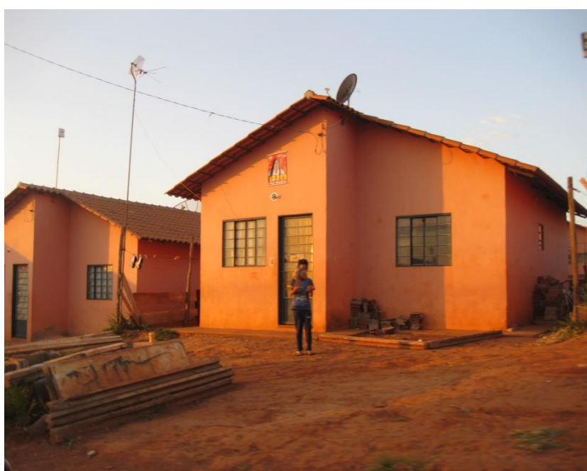
Figure 12 Social houses of the project welfare project “Minha Casa, Minha Vida” (My House, My life).
