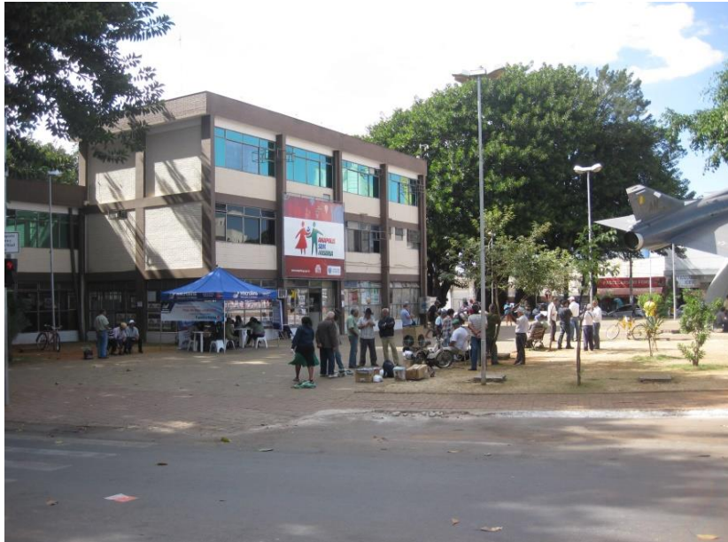
Figure 11 The Square next to the bus station and very close to the Reference Centre for Women. The building in the picture is occupied by other governmental offices of the Secretary for Social Development. On the right, it is visible the back of a military airplane, as Anapolis is the location of one of the most important air force base of the country. Apparently, in this Square there is a lot of semi-hidden prostitution.
