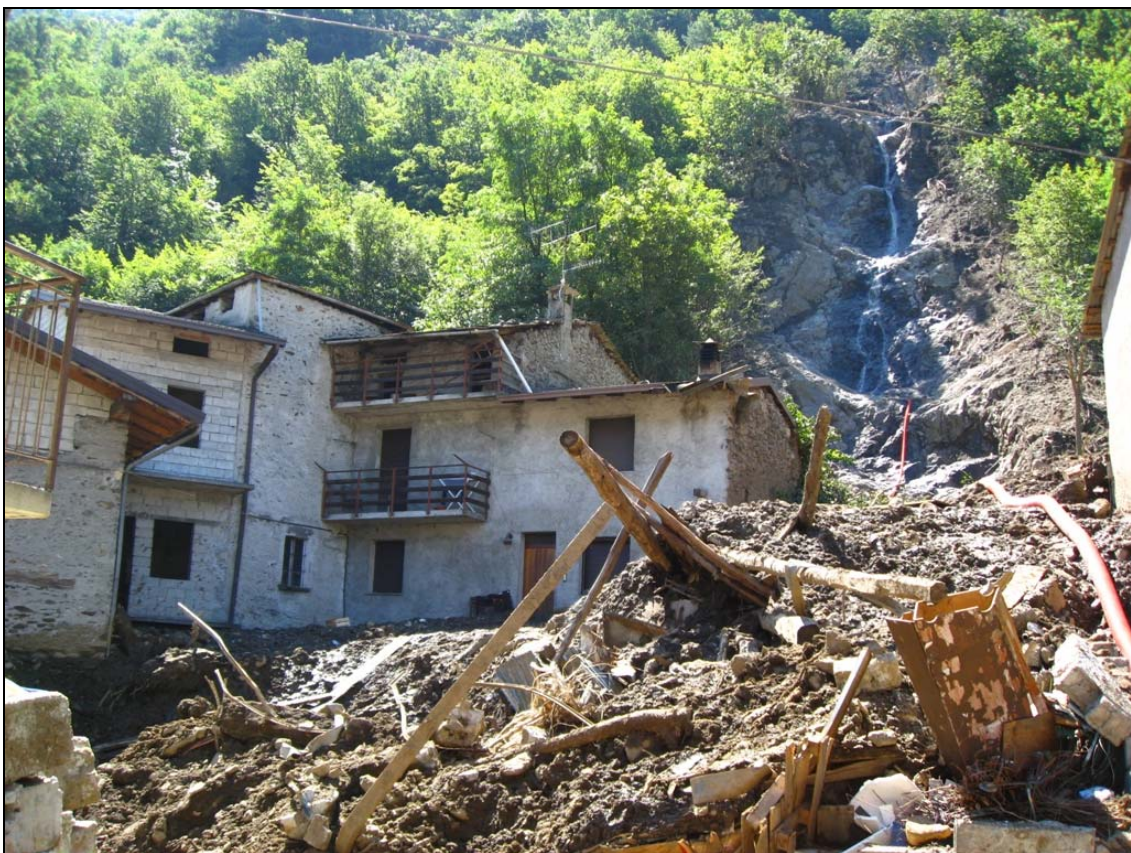
Fig. 10.11 – Remnants of the destroyed building with completely denuded channel of the debris flow behind. Photo J. Blahut.
