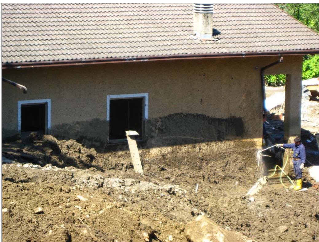
Fig. 10.18 – Building with highest reported damage reaching more than € 290,000. Photo J. Blahut.
