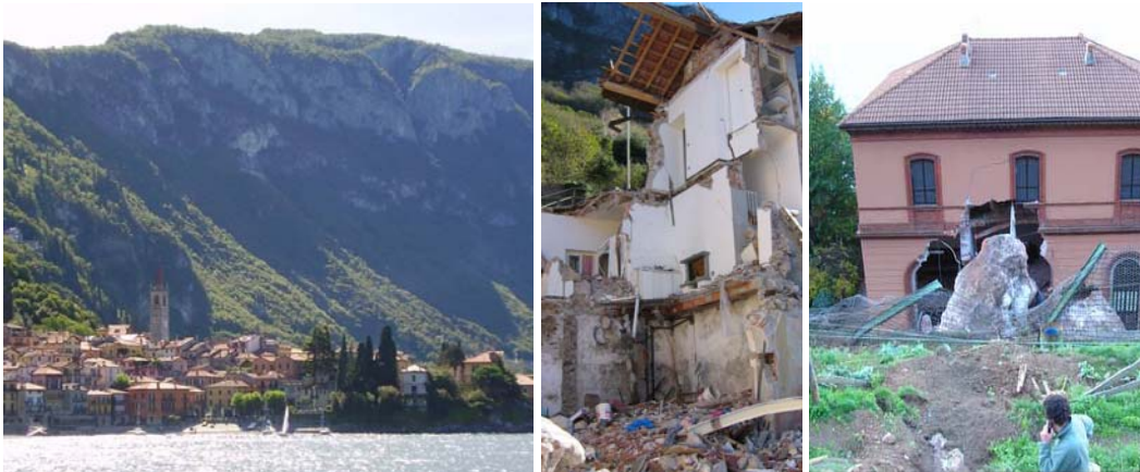
Fig.9. Landslide of Fiumelatte, Varenna (LC). Rockfall occurred on 13 November 2004 and caused 2 casualties and heavy damages to buildings and to railway. A rockfall embankment was realised in extreme urgency conditions. A bigger embankment was designed to protect all the slope of Fiumelatte (in the image on the left)
