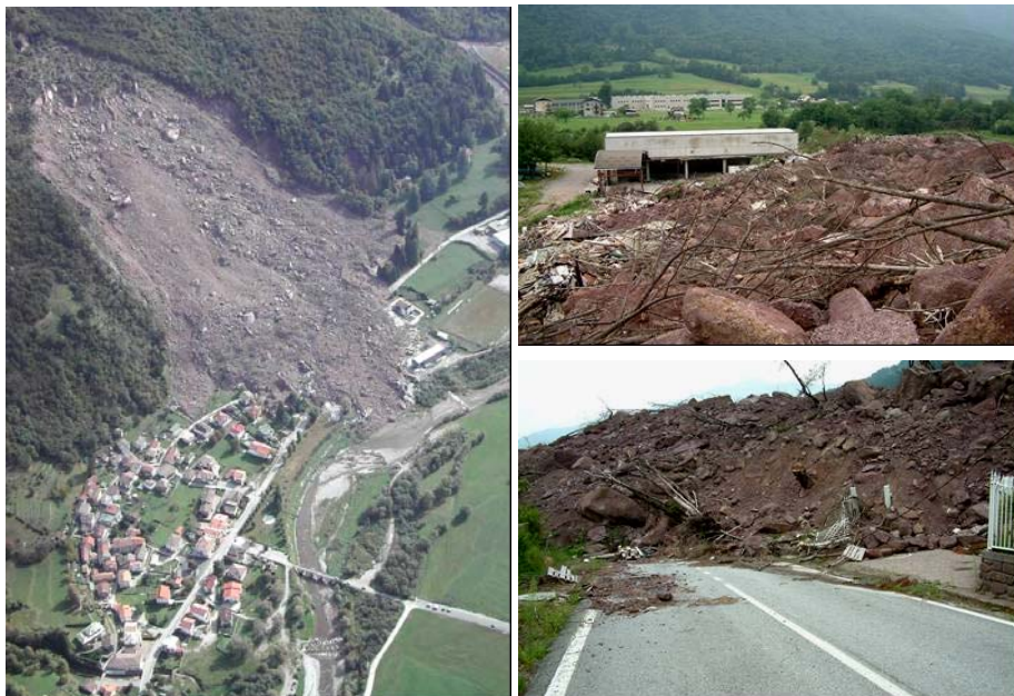
Fig.12. Landslide of Bindo, Cortenova (LC). The event occurred on 1 December 2002. To mitigate the risk connected to the potential reactivation of the instable sectors, a big embankment is designed.
