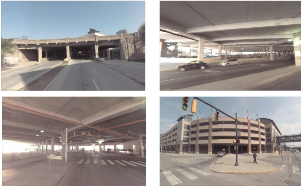
Figure 6.1: Photos of the Virginia Avenue Garage, Indianapolis.
