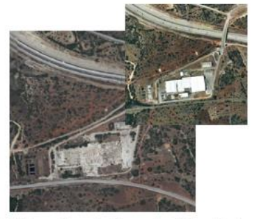
Dismantlement of the regional slaughterhouse
