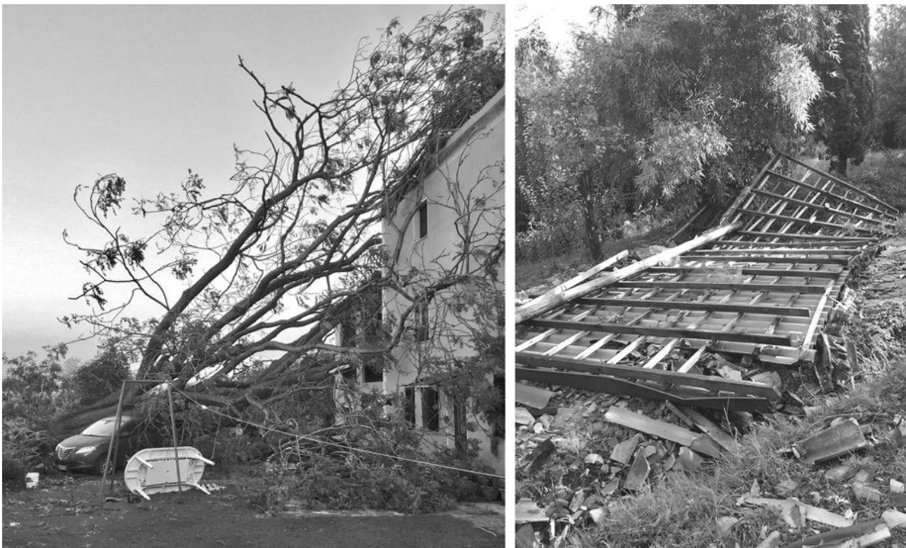
Fig. 24 Damages reported by a interviewee to his holiday house during summer 2020. A violent storm uprooted the historic tree in the courtyard, causing damage to the roof and facade of the building.
