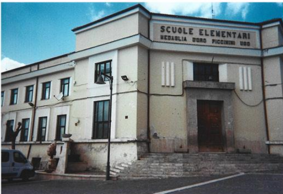
Image 96_4.2 - Barisciano, ex-scuola, photo by A.
