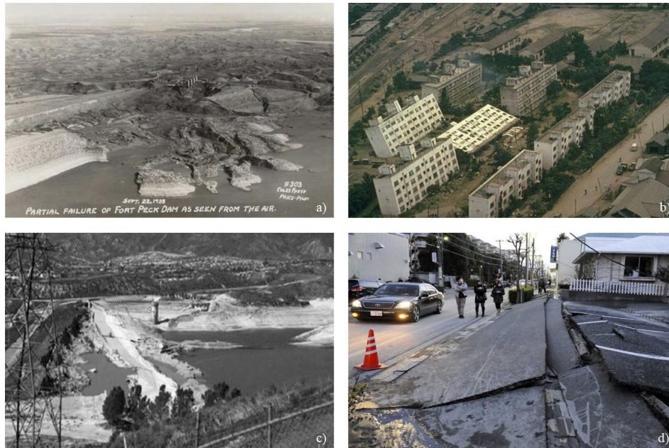
Fig 1.1 Example of liquefaction effect and damages: a) Fort Peck Dam - USA (1938); b) Niigata – Japan (1964); c) Lower San Fernando Dam - USA (1971); d) Japan earthquake 2011
