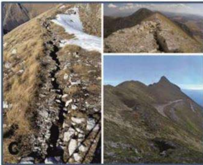
Figure 5 - Fracturing and ground cracks.
