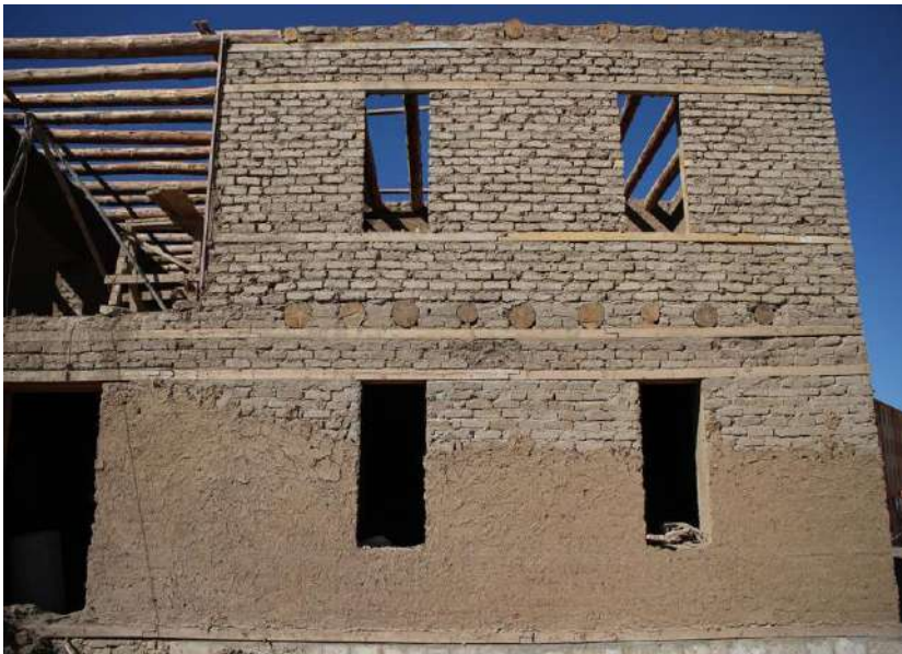
Figure 3 - Adobe house with anti-seismic presides
