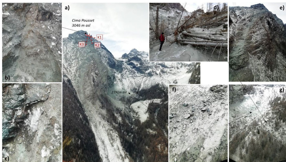
Fig. 2 Pousset peak (a) view with source area; the three main fracture sets controlling the detachment scar, the transit, and the deposits. Three areas with different block depositional characteristics are shown (D1, D2, and D3); (b) source area of the 8300 m 3 rockfall; (c) ice layer along the upper sector of the detachment plane; (d) tree cluster uprooted and covered by a thick dust layer; (e) upward view of the slope; (f) and (g) tree stumps and uprooted trees in the area of thick dust cloud and blocks propagation
